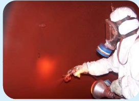
internal lining with food grade coating
