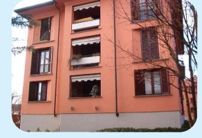
insulation of facades
