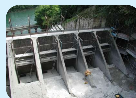
water dam maintenance
