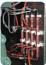
piping and fittings coating
