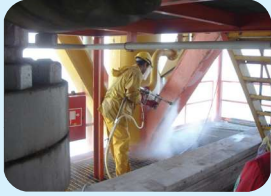
UHPW maintenance works
