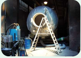
internal lining of vessels
