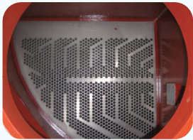
tubesheet and water box renovation
