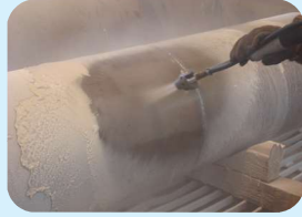
hydro-blasting with non metallic water soluble media
