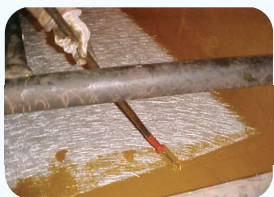
tank bottom rehabilitation
