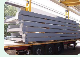
passive fire proofing before erection
