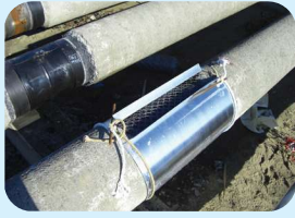
field joint coating
