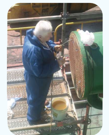
heat exchangers inspections
