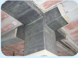
carbon fiber structural reinforcement
