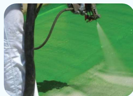
elastomeric membrane waterproofing
