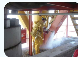
UHPWJ maintenance works
