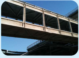
cellulosic fire proofing
