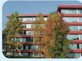
office building maintenance and renovation
