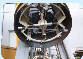
automatic internal blasting and lining
