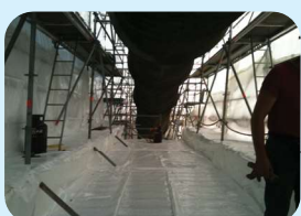
external coating in confined space
