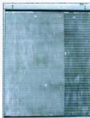
Same units after proprietary abrasive cleaning.
