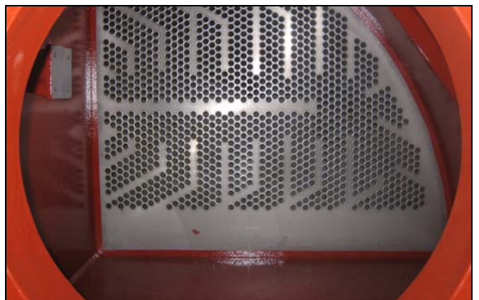
On-site lining of condenser water-box with cold-cured, high-thickness product.
