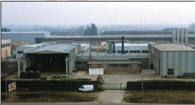
Cuggiono facility: surface preparation and painting shop.
