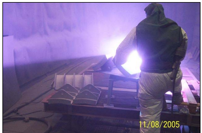
Arc spray zinc metalizing in our shop.
