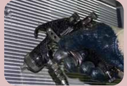
coil protection with bacteria and fungi resistant coatings
