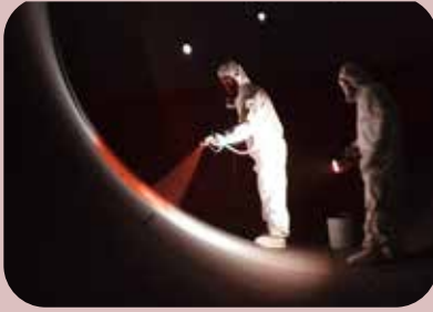
internal lining of tanks with food-grade system
