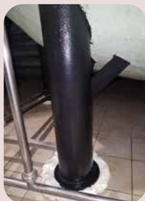
inspections and restorations on external coatings
