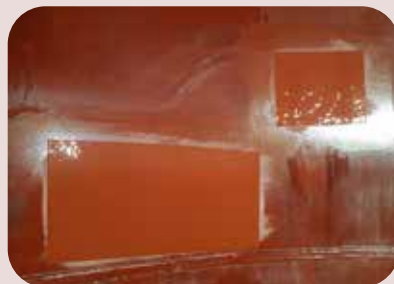
inspections and restorations on interior linings
