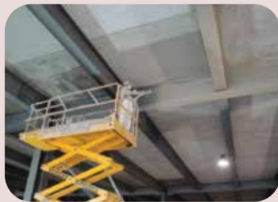
passive fire proofing coating
